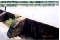
Cracking and deterioration along concrete buttress. Vegetation growth extending from buttress.
