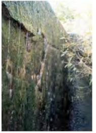
Cracking and deterioration in gunite overlay along buttress wall.
